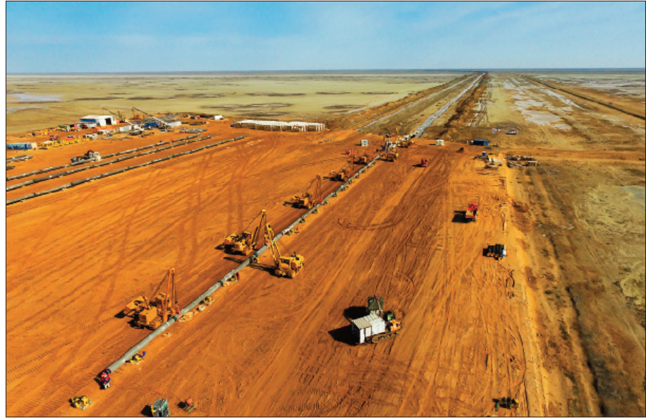
KAZAKISTAN BONATTI Kashagan Pipeline Replacement Project
