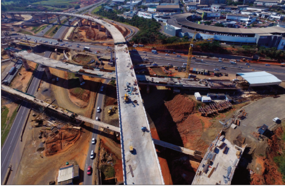
SUD AFRICA CMC Mount Edgecombe Interchange
