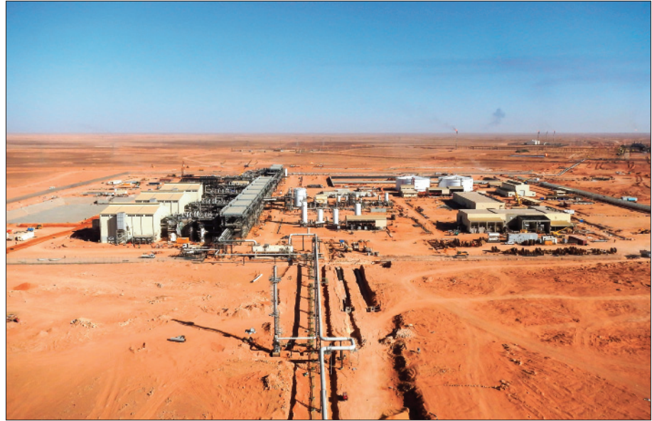
ALGERIA BONATTI Alrar Separation and Boosting Plant
